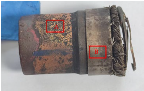
Figure 2. Corrosion sample of air conditioning copper tube. Source (s): Authors' own work
