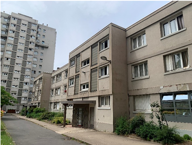
Figure 2. Case study site: 1950s Paris social housing complex
