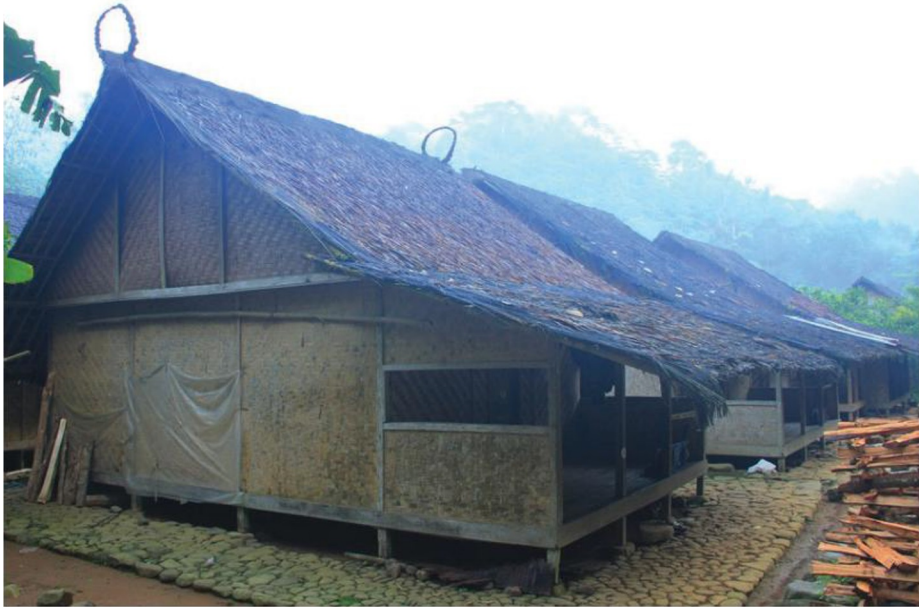
Figure 4. The Baduys' house: the designed roof to slip volcanic ash to the ground Source: Firdaus et al. (2023)
