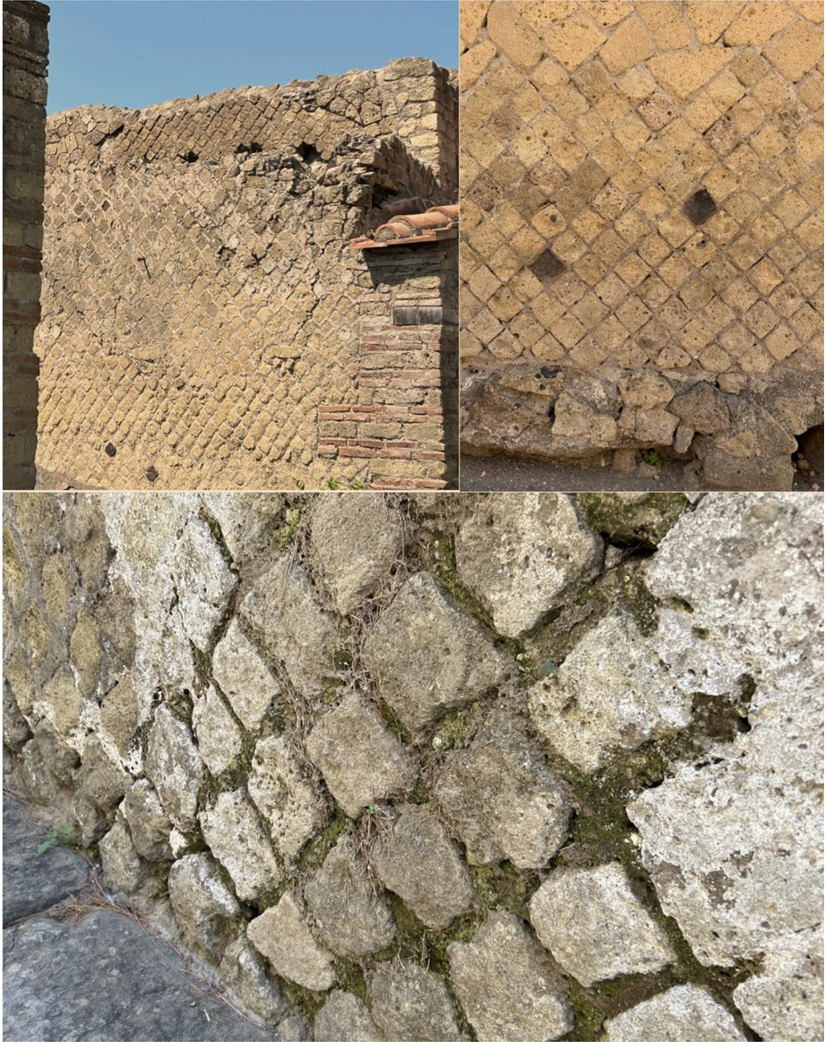
Figure 7. Opus Reticulatum on the house's walls at the archaeological park of Herculaneum, Ercolano, Italy: buried under volcanic ash and pumice in the eruption of vesuvius in 79 AD Source: Photos by Mariana Oliveira (September 9th, 2023)
